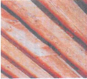
Timber fence cladding
